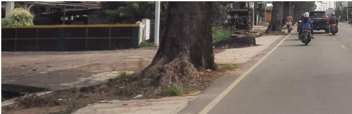
Figure 13. The area around the tree roots has been covered with a layer of cement.
