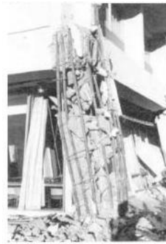
Fig. 11 The failure of reinforce concrete weak column Sources: Website Earthquakes and Earth's Layer
