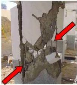
Fig. 9 Diagonal Cracks in Type of a Column Sources: Website Earthquakes and Earth's Layers
