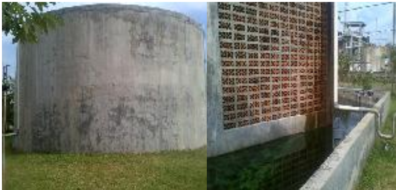
Figure 4. The 700 cubic m of anaerobic digester
