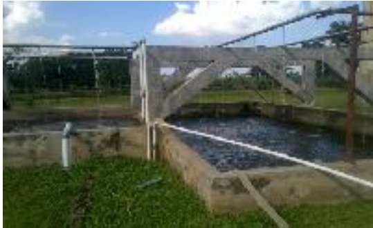
Figure 2. The aeration pool
