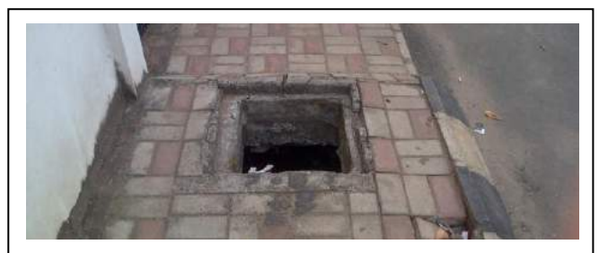
Figure 3. Drainage Hole Source: Author
