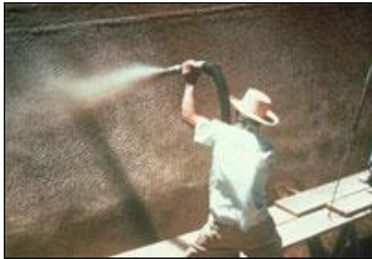
Figure 1.1. Shotcrete application
