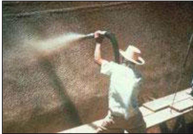
Figure 1.1. Shotcrete application
