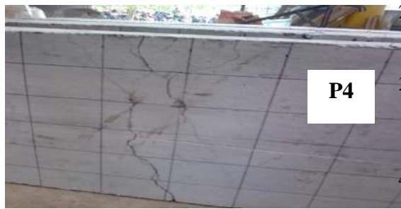
Figure 9: crack pattern test specimens
