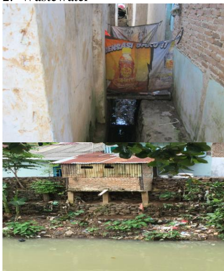
Figure 19. Sewerage citizens Jembatan Beton Way Blau [10]
