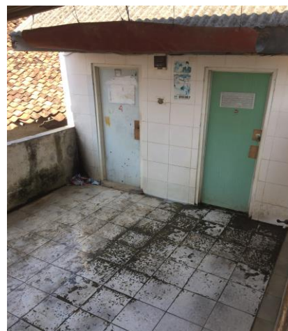
Figure 18. Toilet Kampong Jembatan Beton Way Blau [10]
