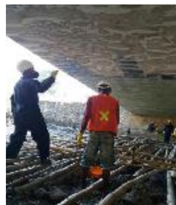
Figure 6. Strengthening bottom slab of box-girder bridge using GFRP Tyfo SEH51A composite
