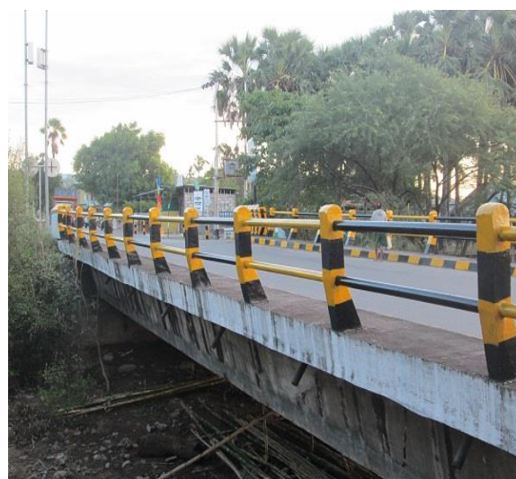
Figure. 2 Namosain box-girder bridge lay near the sea.
