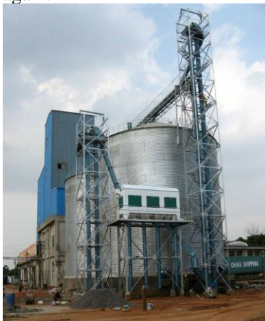
Figure 4. Steel Grain Storage Silo
