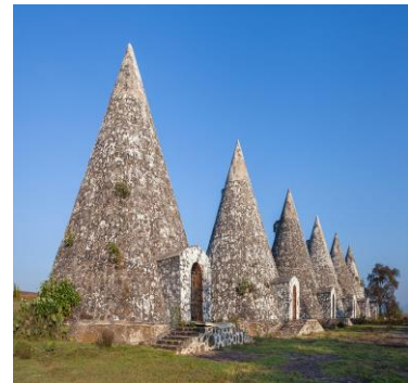
Figure 3. Traditional SILO in Mexico
