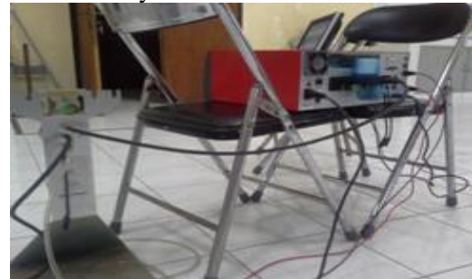
Figure 2. Generator Exhaust Emission Testing Front with 898. Stargas tool Installation
