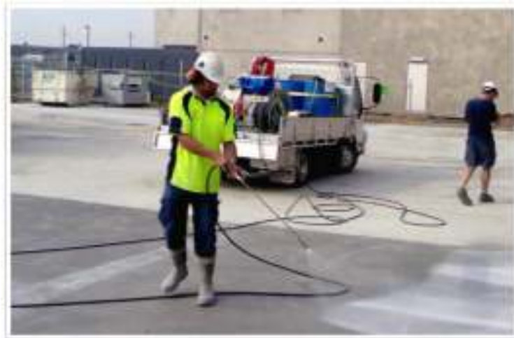
Gambar 3.1 Curing compound secara manual
