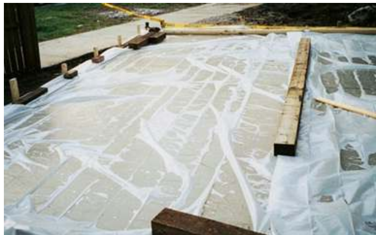
Gambar 3.3 Waterproof curing
