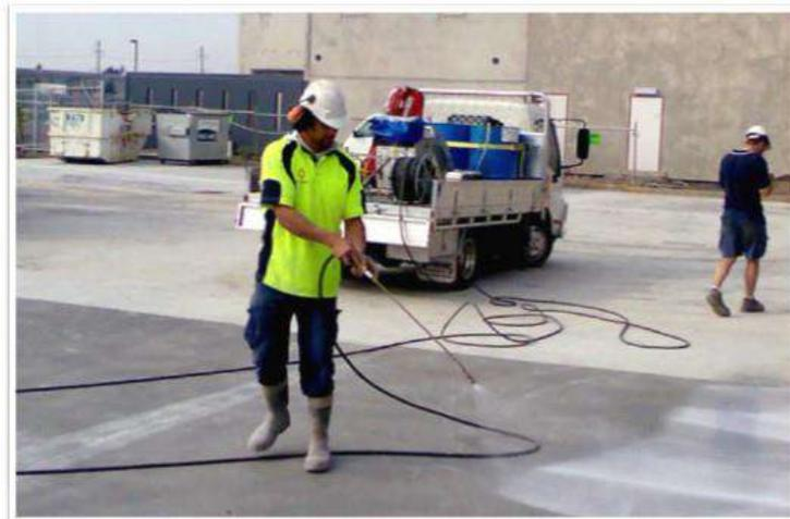
**Gambar 3.1 Curing compound secara manual**
