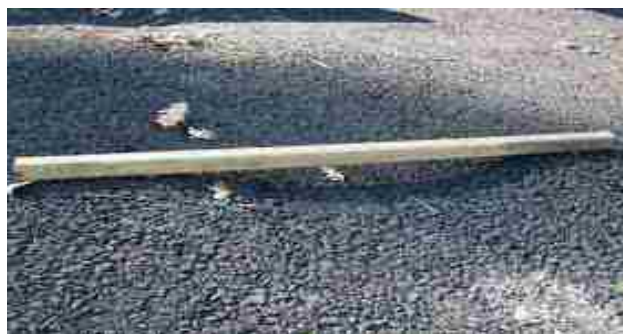
Gambar 2.8. Kerusakan Polished Aggregate
